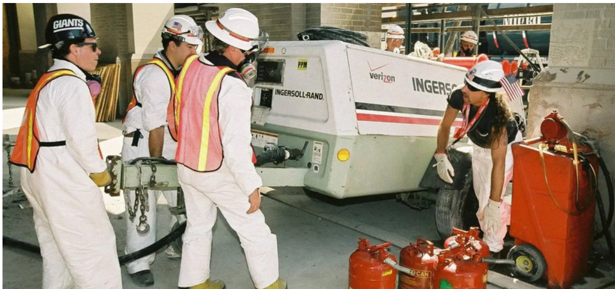
Technicians bring in air compressors. Everything had to be rebuilt.
