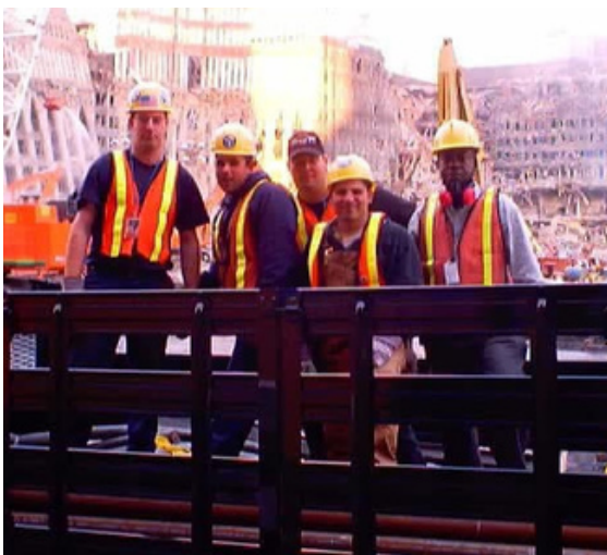
ECS workers were working at Ground Zero from Day 1
