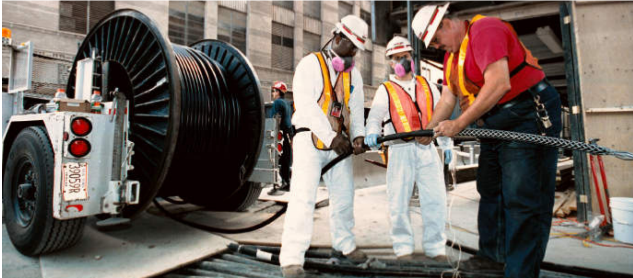
Line gang and CXM techs preparing cables to run along the sidewalk to restore service quickly
