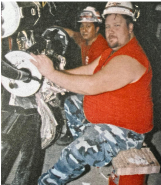
Cable splicers Bobby Chew and Tommy Schaeffer in the vault at 140 West St. This photo appeared in the NY Generator one year anniversary issue October 2001.
