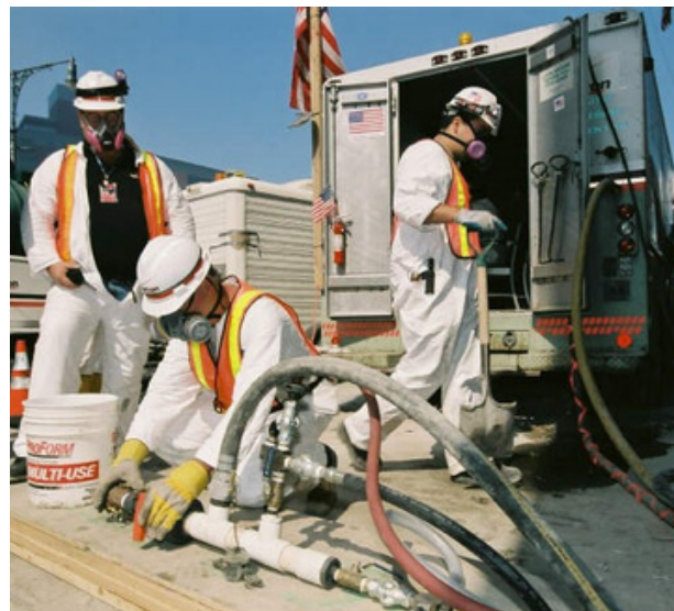
Techs put air pressure on the cables to keep water out
