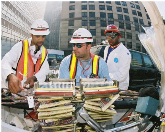
Every 3600 pair cable had to be respliced.
