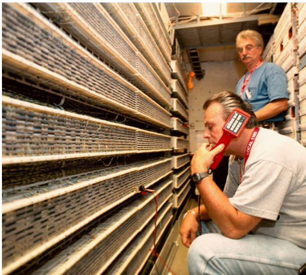
Local 1101 members worked inside and outside to restore service
