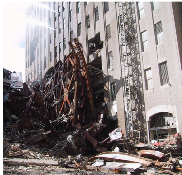
The damage to 140 West St was extensive
